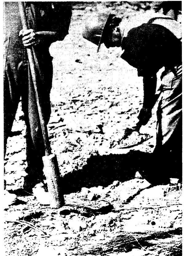
Photo 35.5. Tamping blastholes.
