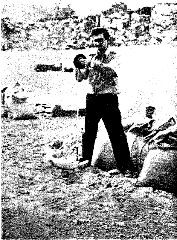
Photo 35.3. Flexible measuring tape to control charge height and blasthole depth.
