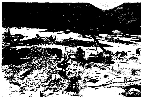
Photo 34.3. Placing of a heavy covering upon a small blast.
