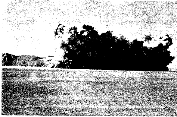
Photo 33.1. Alterations produced by blasts: vibrations, air blast, fly rock and dust.
