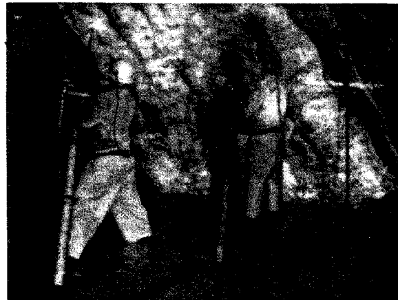
Photo 22.2. Manual drilling in a drift face.
