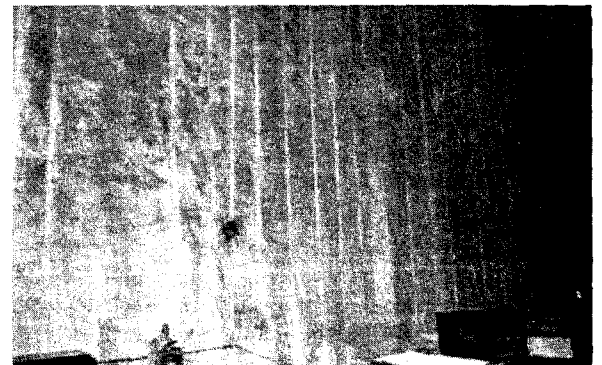
Photo 24.4. Side walls with presplitting in the Hydroelectric Power Station of Saucelle (Iberduero, S.A.).
