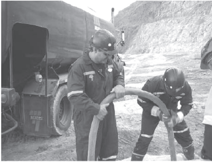
Figure 25.4 Lowering of slurry explosive hose to the bottom of the blasthole.
