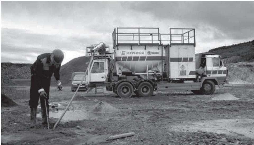
Figure 25.3 Truck for charging a blasthole by slurry explosive.
