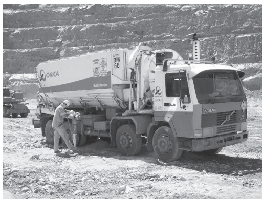
Figure 25.1 Charging of a blasthole by use of explosive mixed by a delivery truck.
