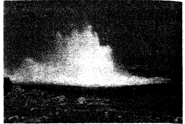
Photo 26.1. Underwater blasting
